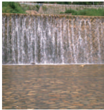
Upper Reaches of Sumiyoshi River
